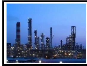
Complex Oil Refinery
